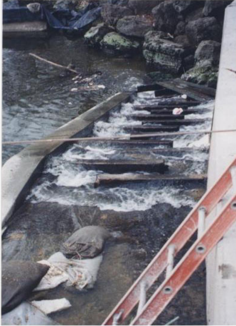
Figure 20. Existing ‘fishway’ at the west bank of Kimball Street Dam in Elgin, Illinois. Reasons for failure to pass fish include: insufficient attraction flow, too steep, insufficient pool size (no energy dissipation), excessive water velocity, and insufficient depth.
